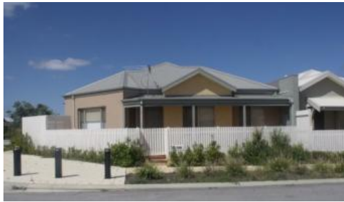
46A Salterforth Road St, Butler
